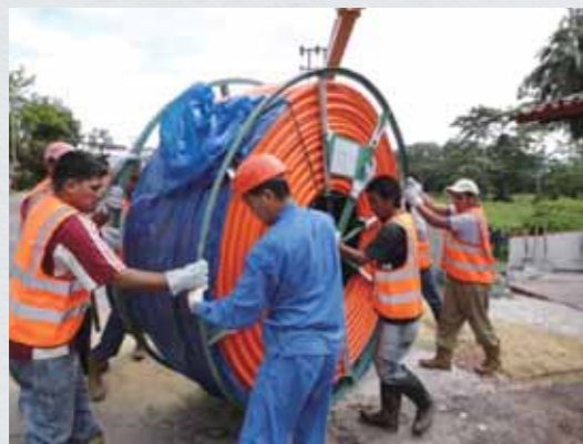
Overseas construction site
