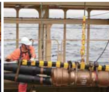
Submarine cable construction
