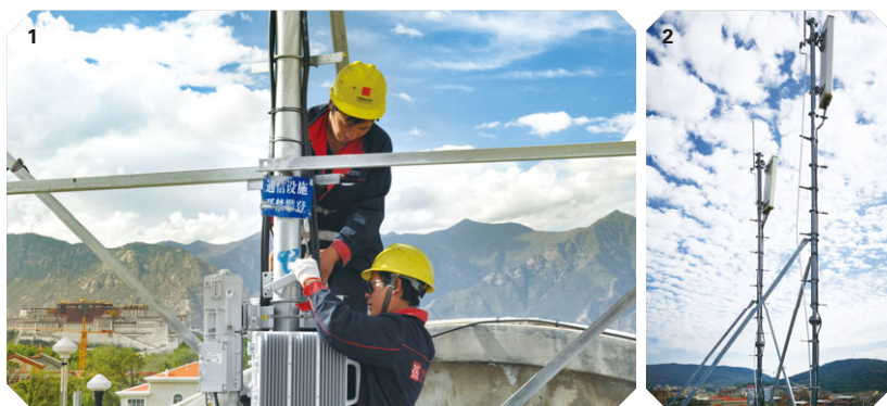
1 & 2. The Group undertook construction of telecommunications network and 5G project
