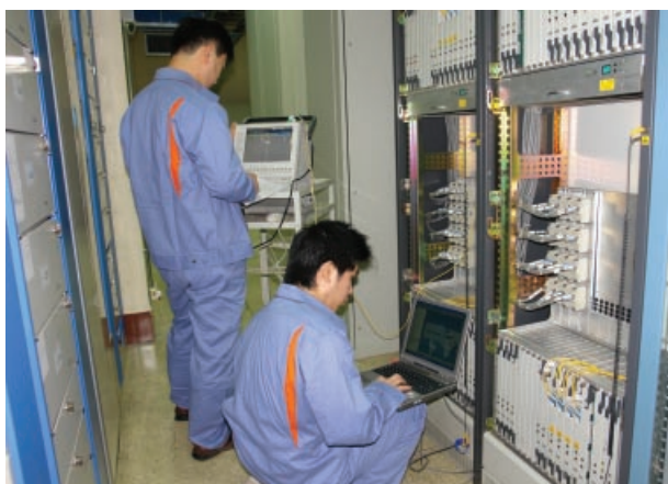
Tuning and testing of transmission equipment for the machinery room at Baiyuan Airport, Guangzhou
