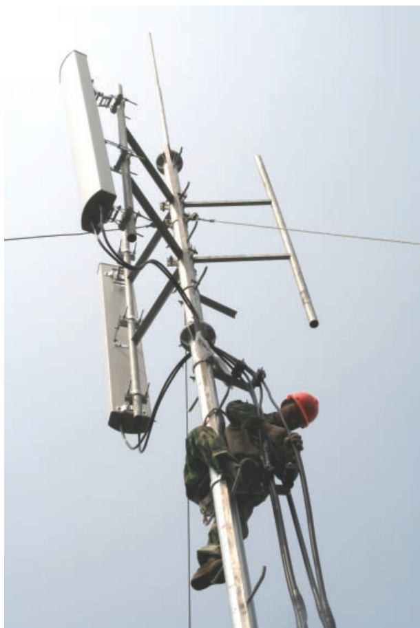
Construction of mobile base station
