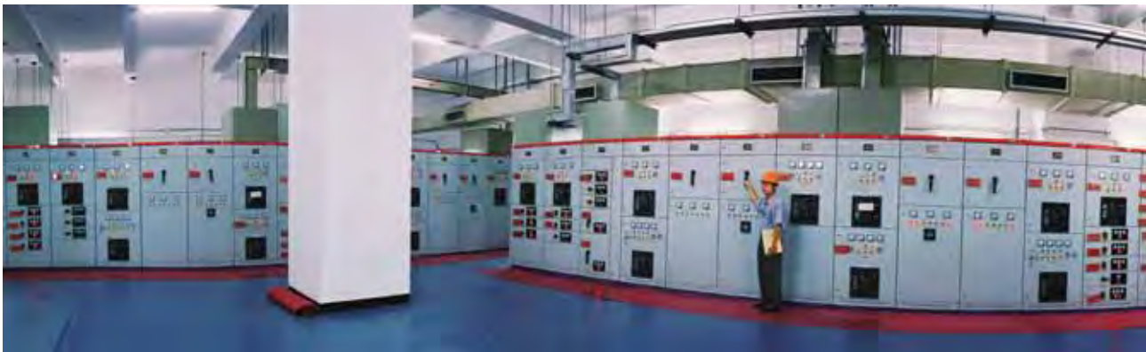
☉ Equipment installation quality checking
