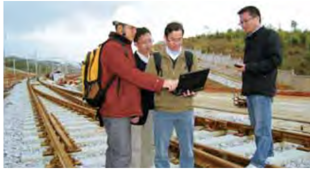
☉ Design staff carried out testing of wireless communication in Wuhan-Guangzhou high-speed railway
