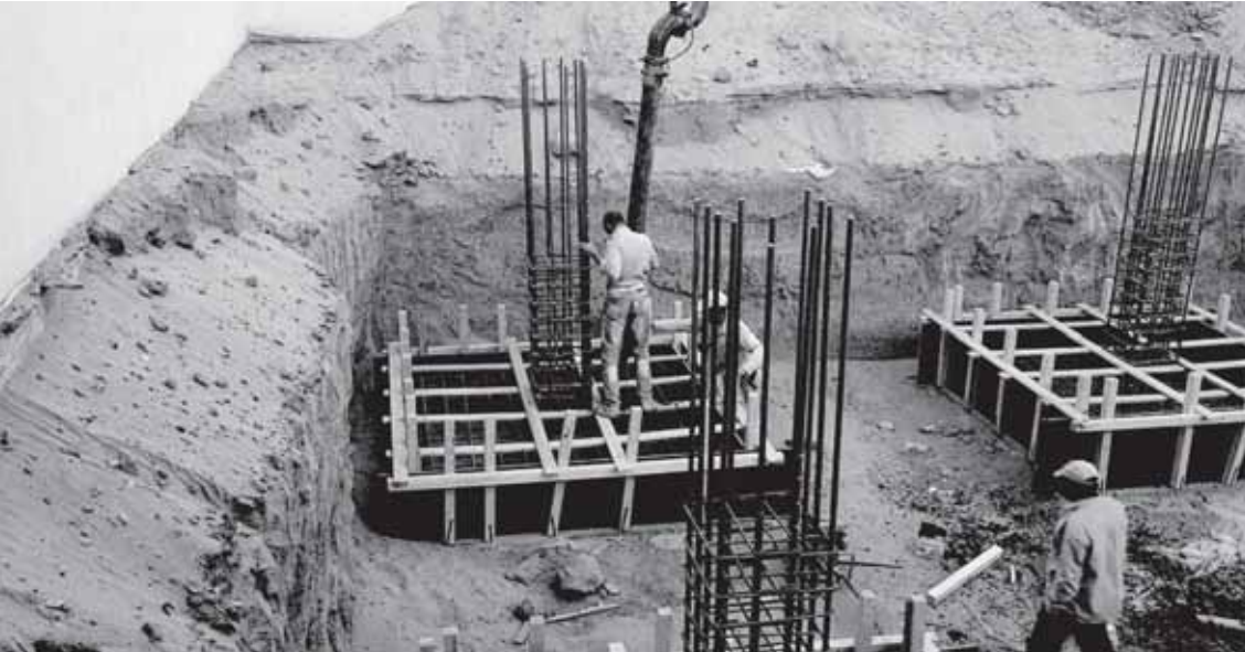
Overseas Construction Sites
