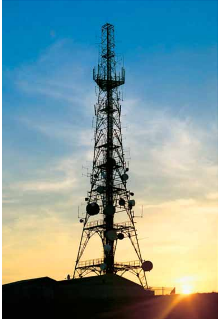
Base Station Maintenance Projects
