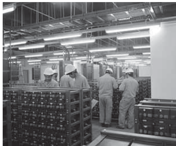
Fiber optic broadband network project in the information park
