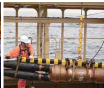
Submarine cable construction
