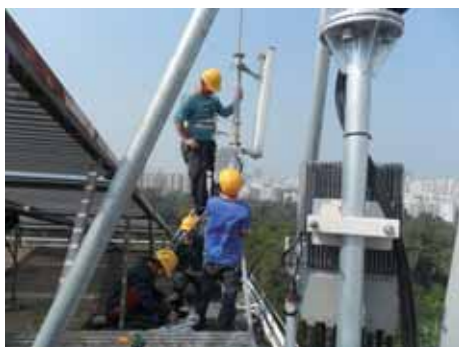
4G equipment installation and base station construction
