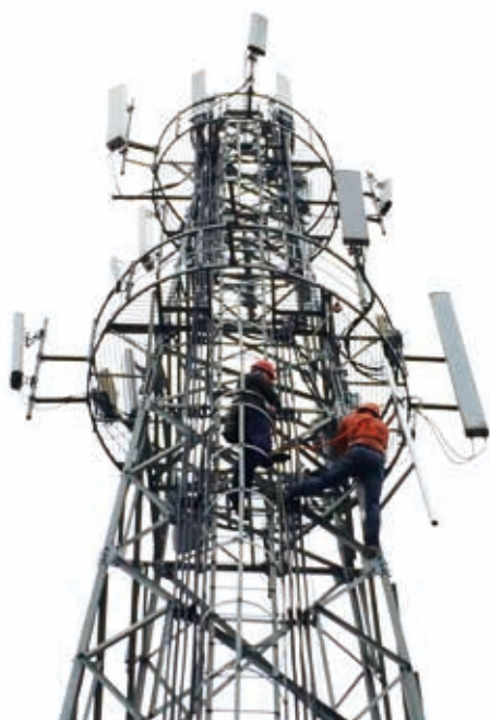
The Group undertook integrated construction and maintenance projects of the towers
