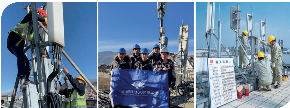
The Group undertook 5G base stations construction
