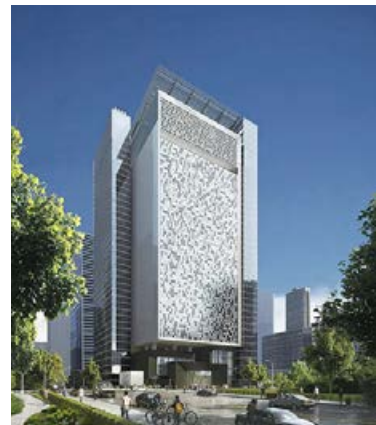
● An Artificial Intelligence Data Center (EPC) Project in Qianhai
