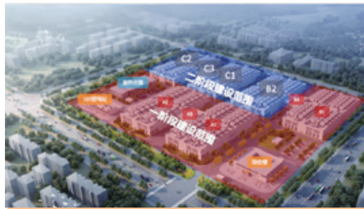
◆ A Leading Internet Company's Intelligent Cloud Ulanqab Data Center Project
