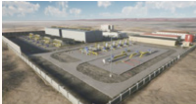
◆ A Gas and Safety Early Warning Construction Project in a County
