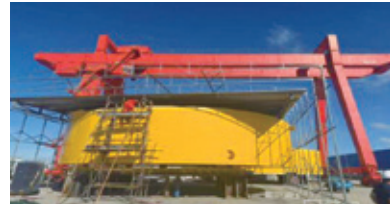
◆ An Underwater Data Server Room Construction Project
